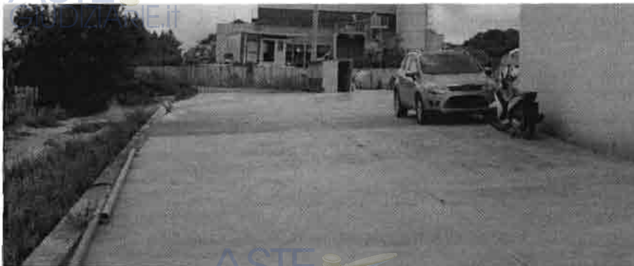
Piazzale in c.a.
