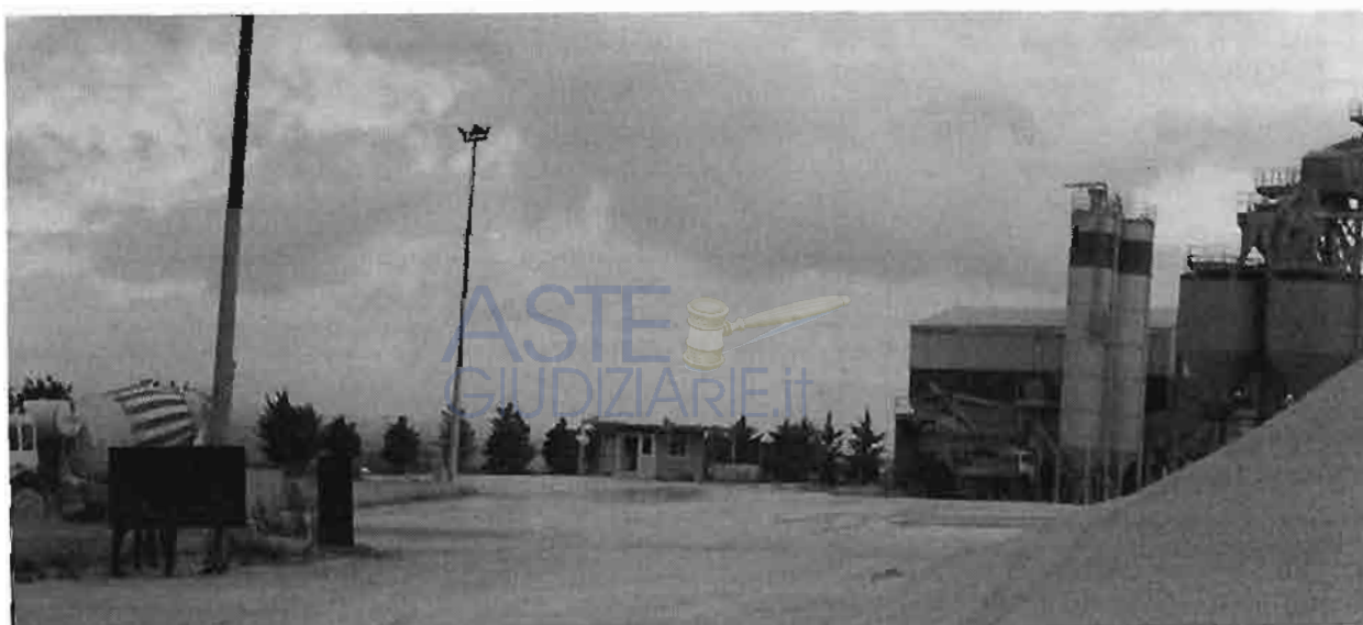
Piazzale in c.a.
