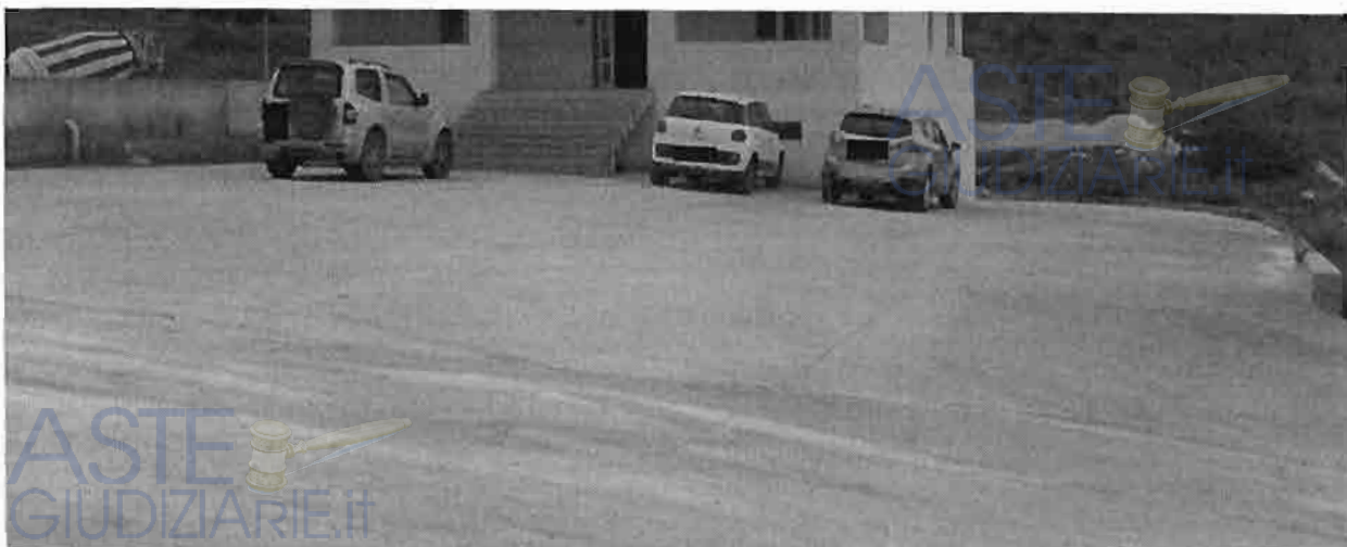
Piazzale in c.a.
