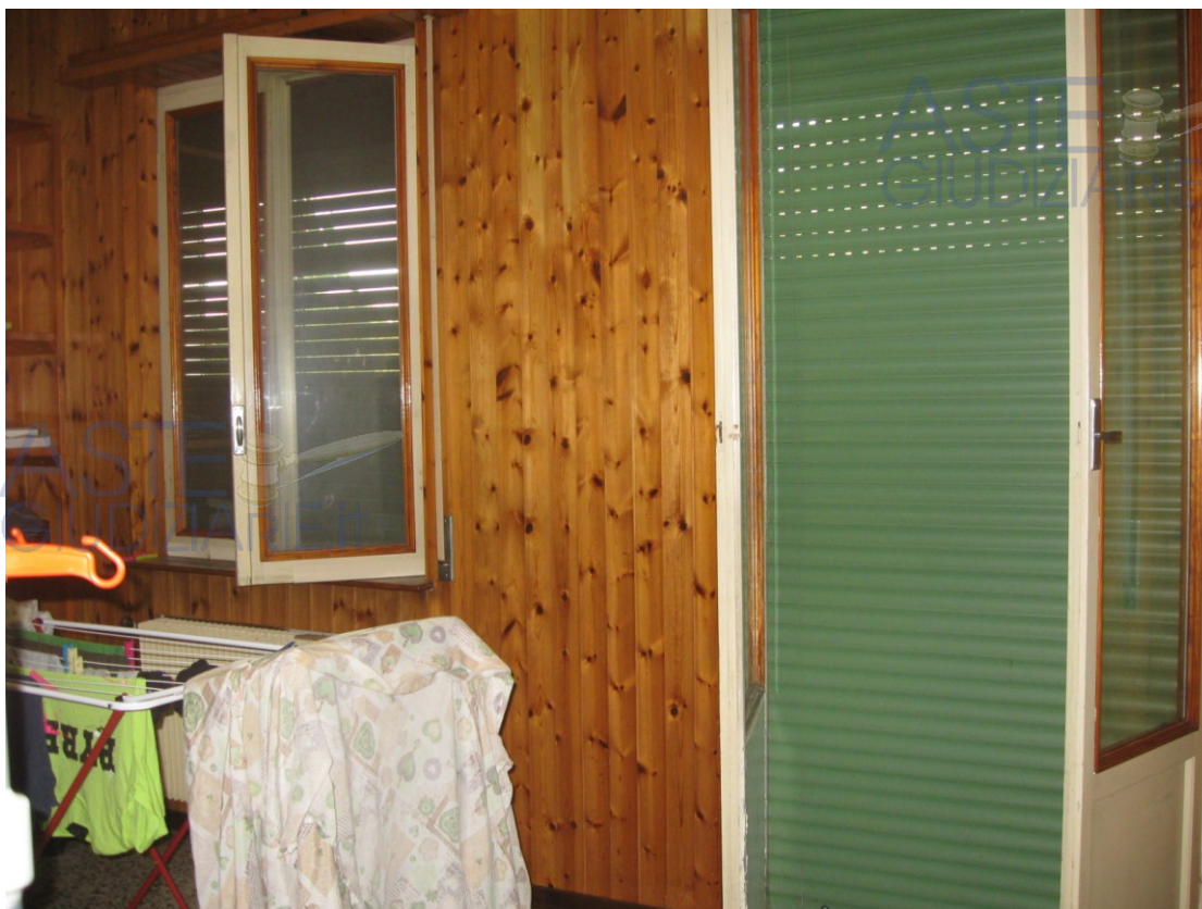
V8 Vista interna camera 1
