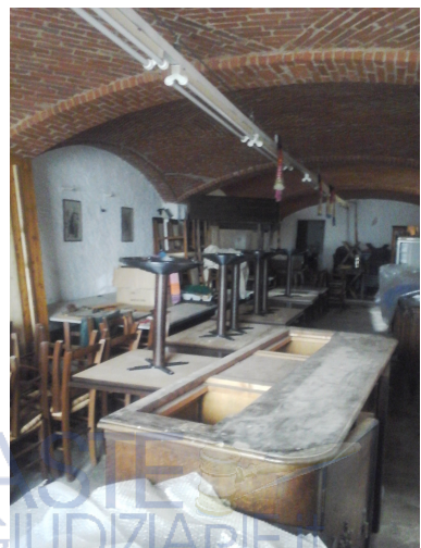
Piano terra – interno locale
