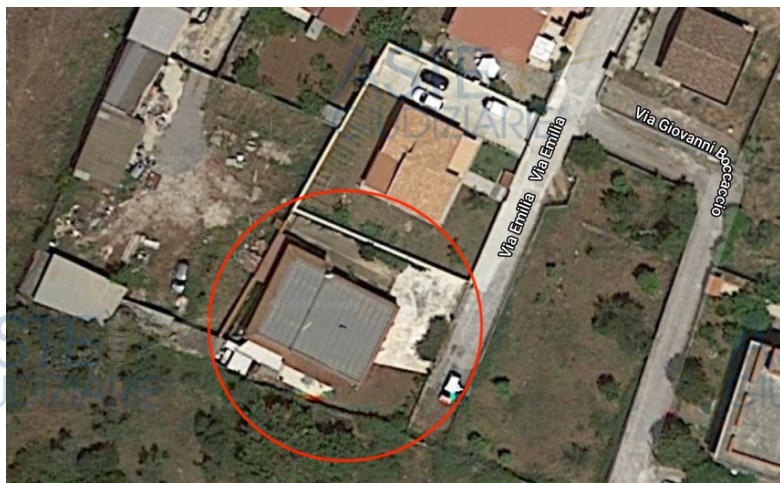
(Foto aerea Google Maps 09/02/2021);
